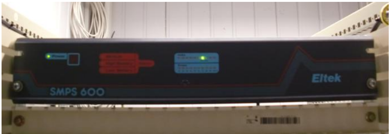
Figur 3-6 Strømforsyning i server-rack.
