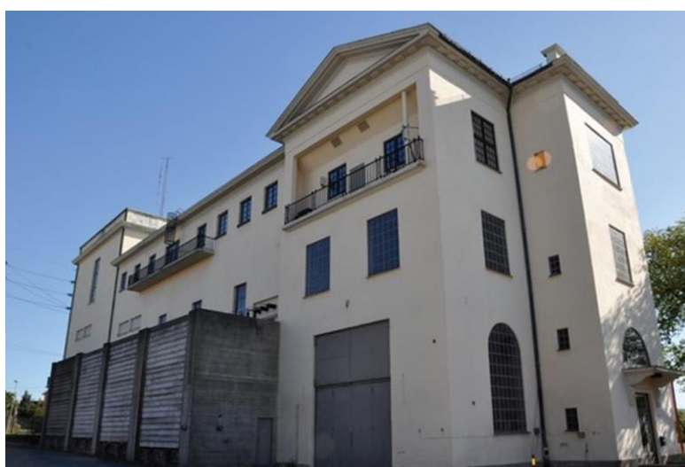
Figure 3 – Substation example of Tonsen substation located in Oslo [6].
